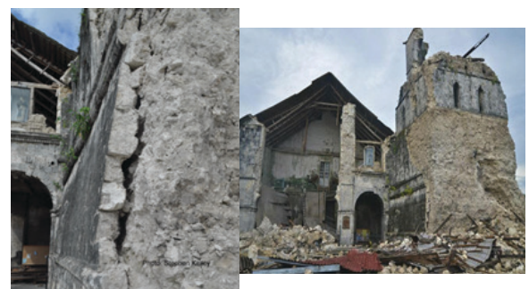
For the Baclayon Church, although the wall dimensions are massive, it appears that there is only some fitted stone masonry cladding that shores up the interior rubble material mostly calcareous rock and sand of weak or no cementation at all. Photographs by Mr. Stephen Kelley (left) and Mr. Anthony Manding (right).
