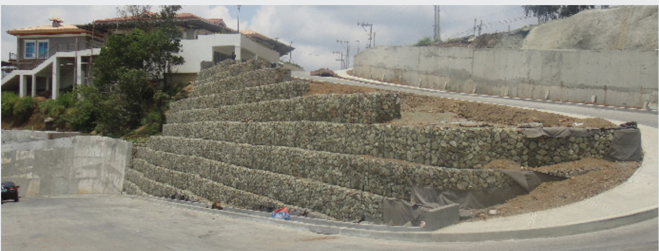
Constructed MSE wall for Twin Lakes Vineyard
