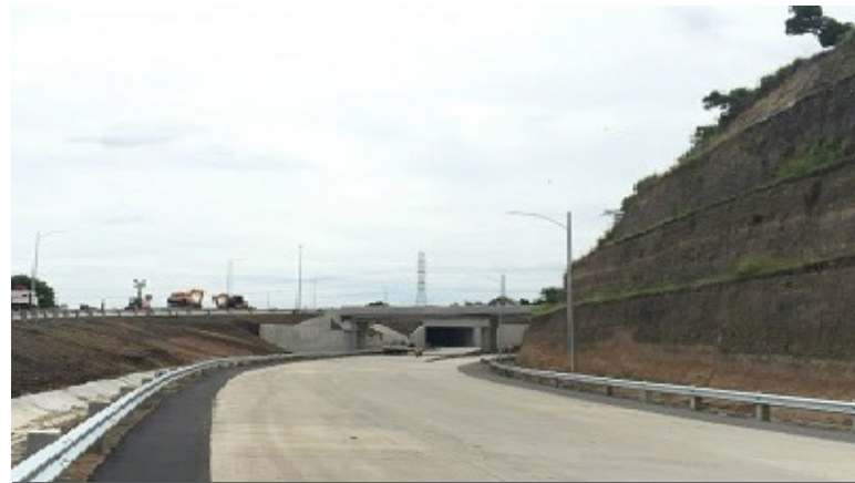
Design of slope protection for the SLEX-Daang Hari Link Road
